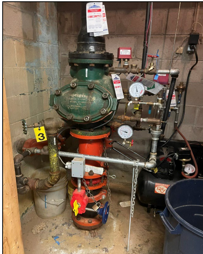
Photo 20: Dry-Type Sprinkler System
