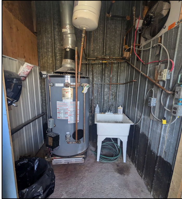
Photo 14: DHW Heaters (Mechanical Room)
