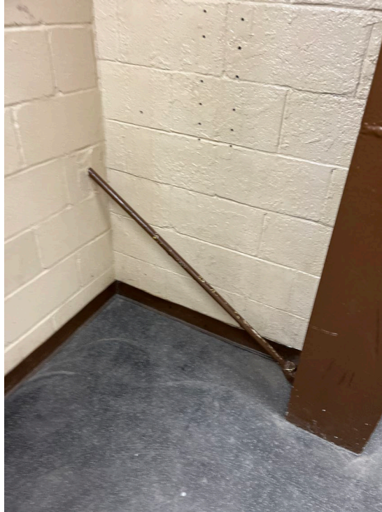
Photo 22: Cross bracing observed to go through concrete block wall.
