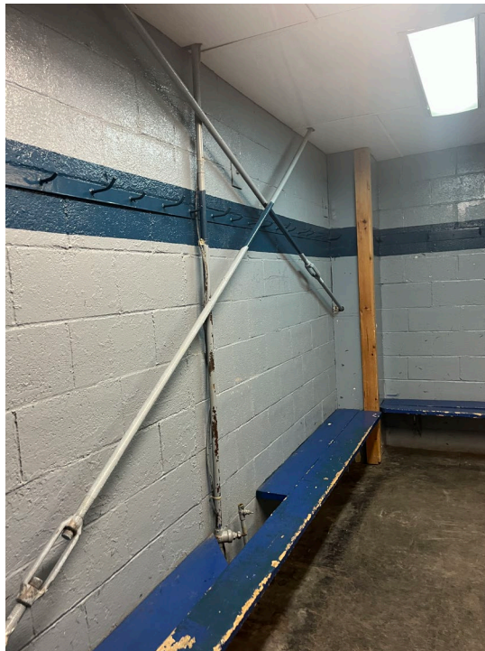
Photo 18: Cross bracing at east side dressing room.
