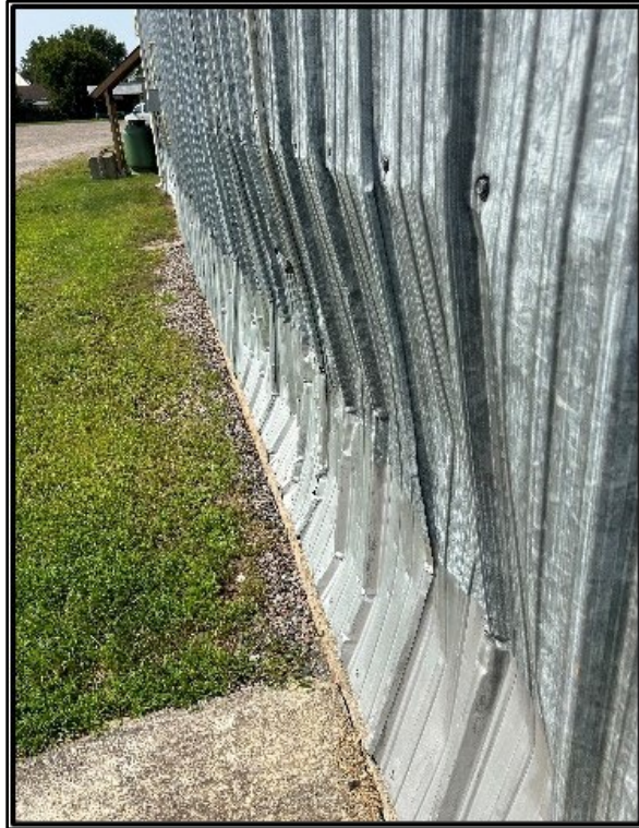
Photo 4: Exterior cladding with visible rusting.
