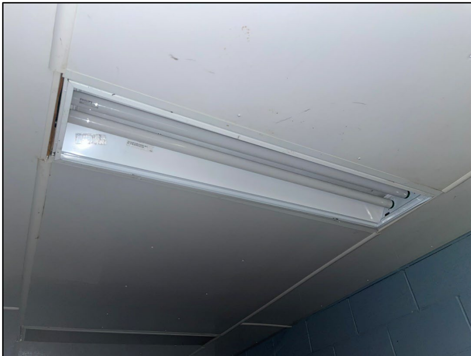
Photo 14: Damaged Lighting Fixtures
