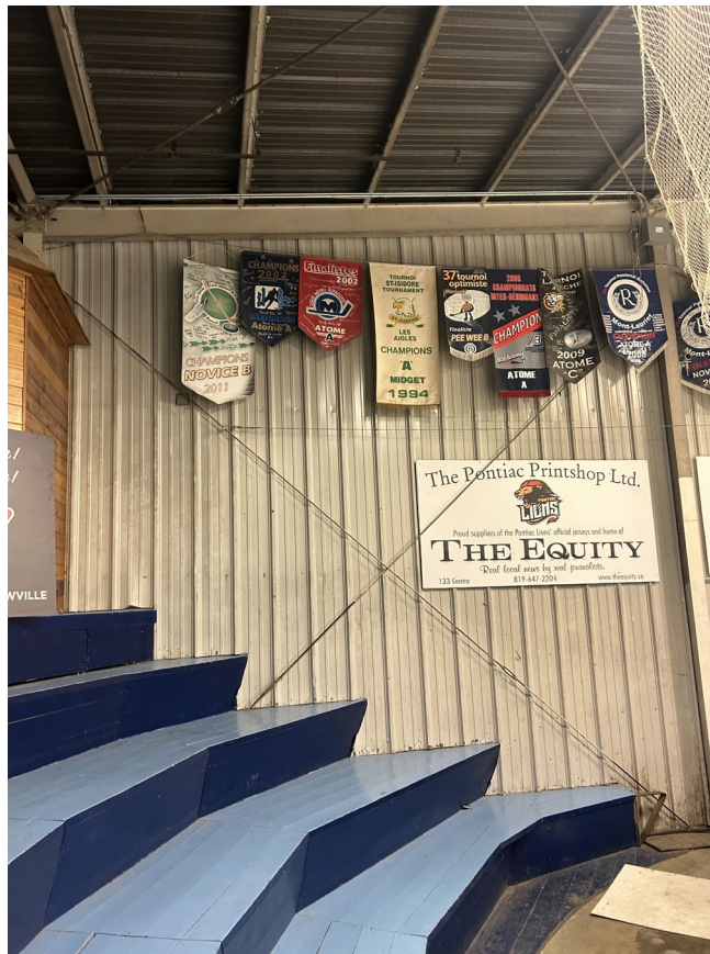
Photo 10: Cross bracing at back wall of arena.
