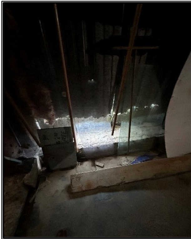
Photo 2: Section loss at exterior cladding seen from inside the structure.
