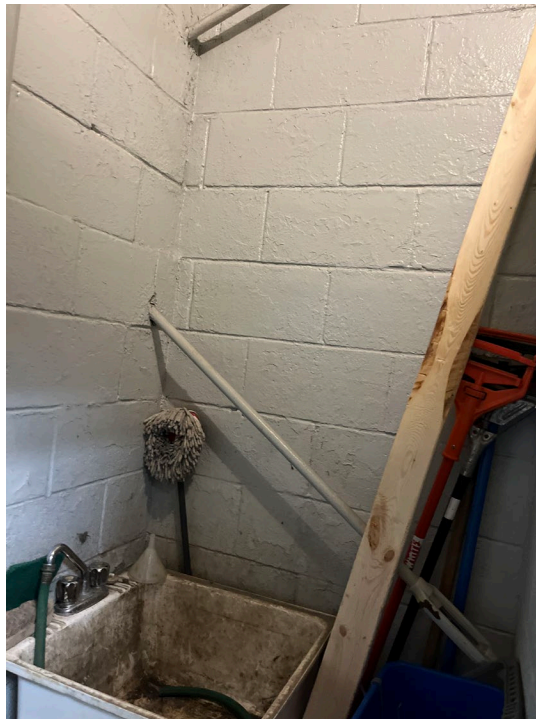
Photo 22: Cross bracing observed to go through concrete block wall.
