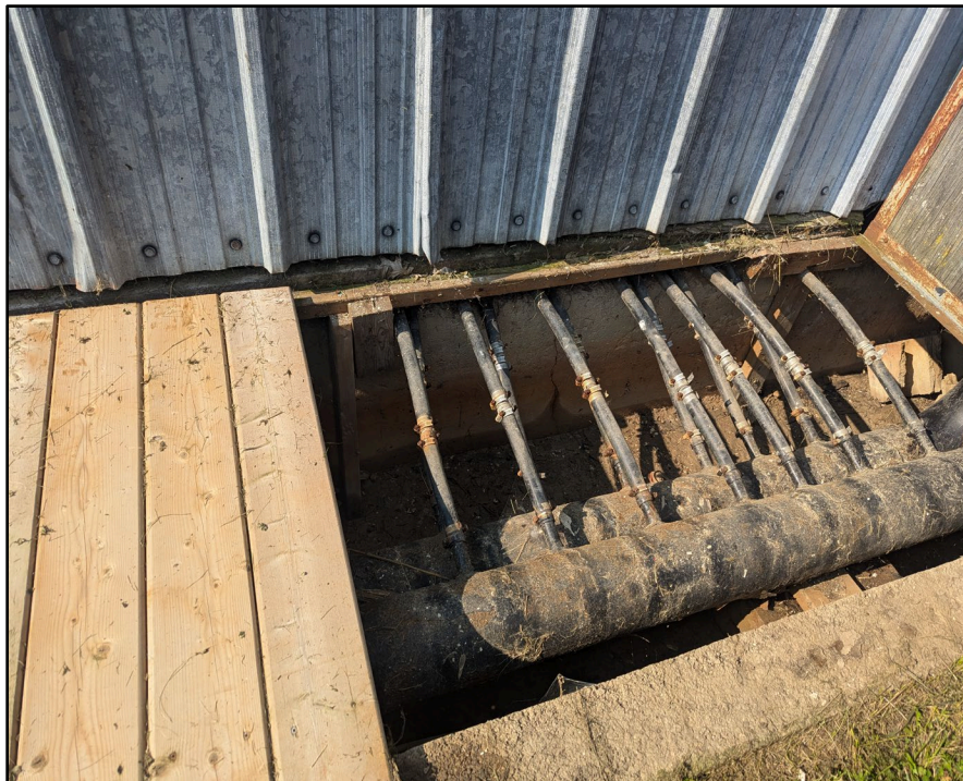
Photo 4: Brine of Glycol Circulation Pipes
