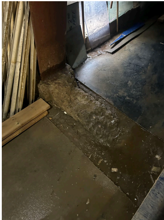
Photo 14: Exposed deteriorated base slab underneath west bleachers.
