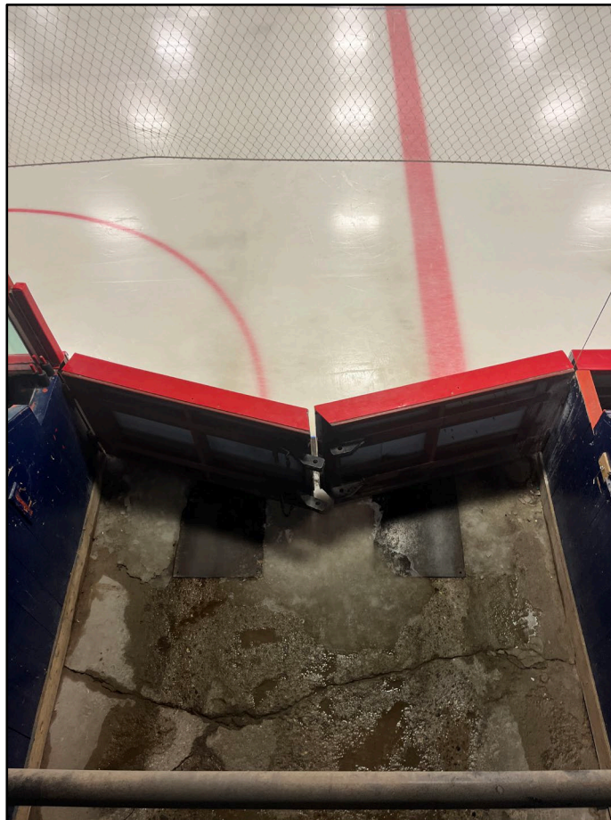
Photo 12: Exposed base slab at Zamboni entrance.
