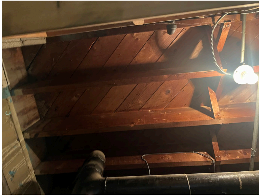
Photo 23: Wood beam elements under mezzanine.
