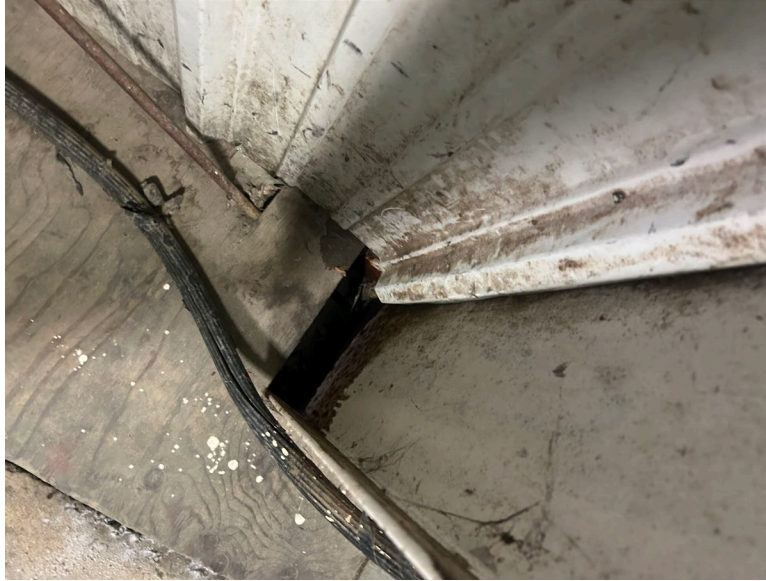
Photo 12: Exposed base slab at Zamboni entrance.
