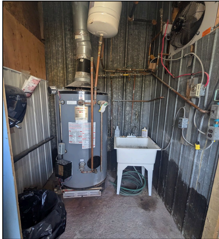
Photo 14: DHW Heaters (Mechanical Room)
