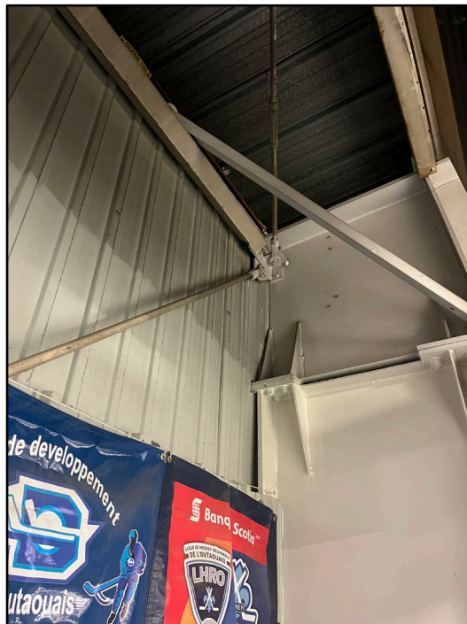
Photo 8: Cross brace connection to steel roof beam at southeast end arena.
