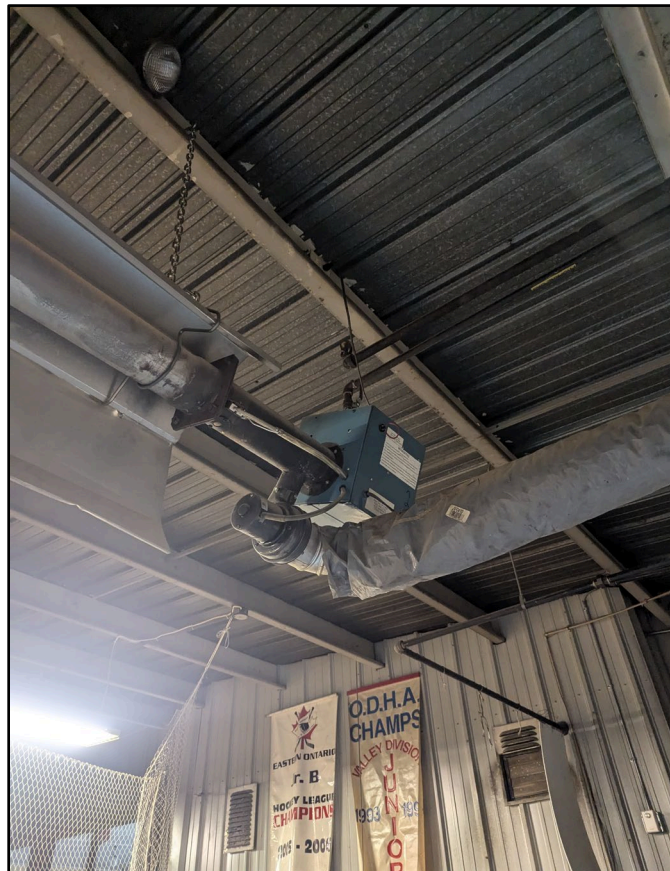
Photo 28: Tube Radiant Heater
