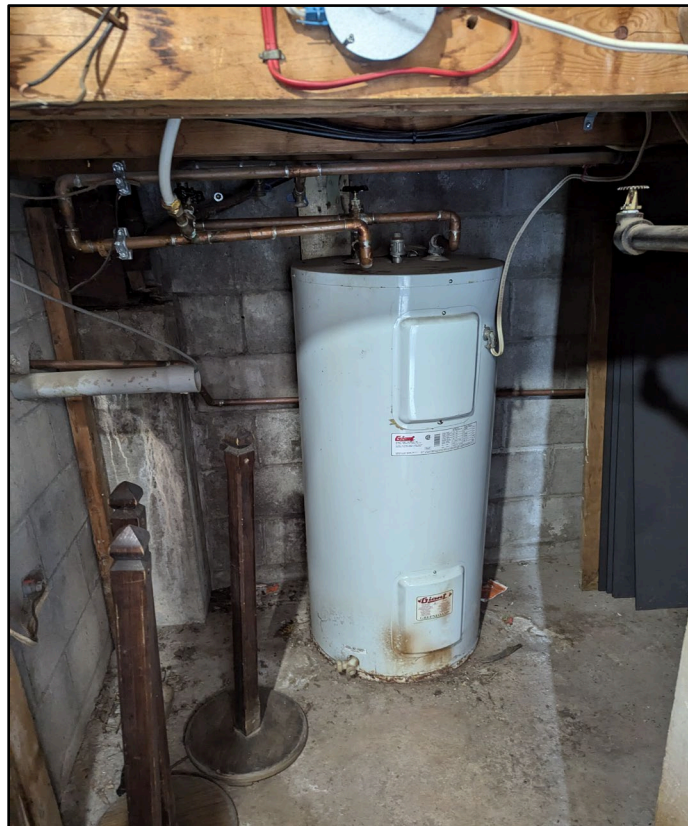
Photo 12: DHW Heater (Stairs)
