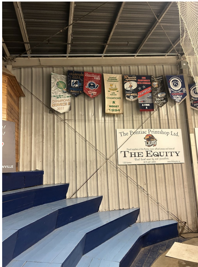
Photo 10: Cross bracing at back wall of arena.
