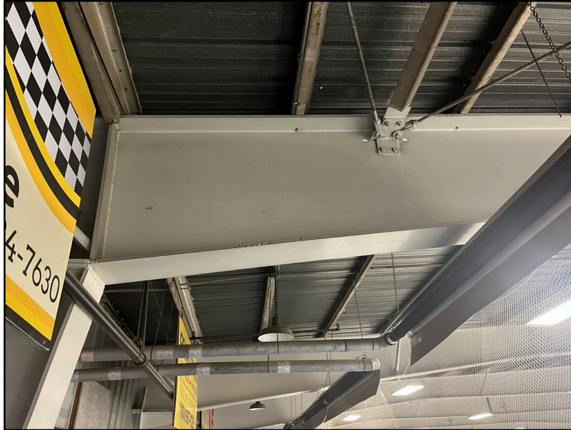
Photo 10: Cross bracing at back wall of arena.
