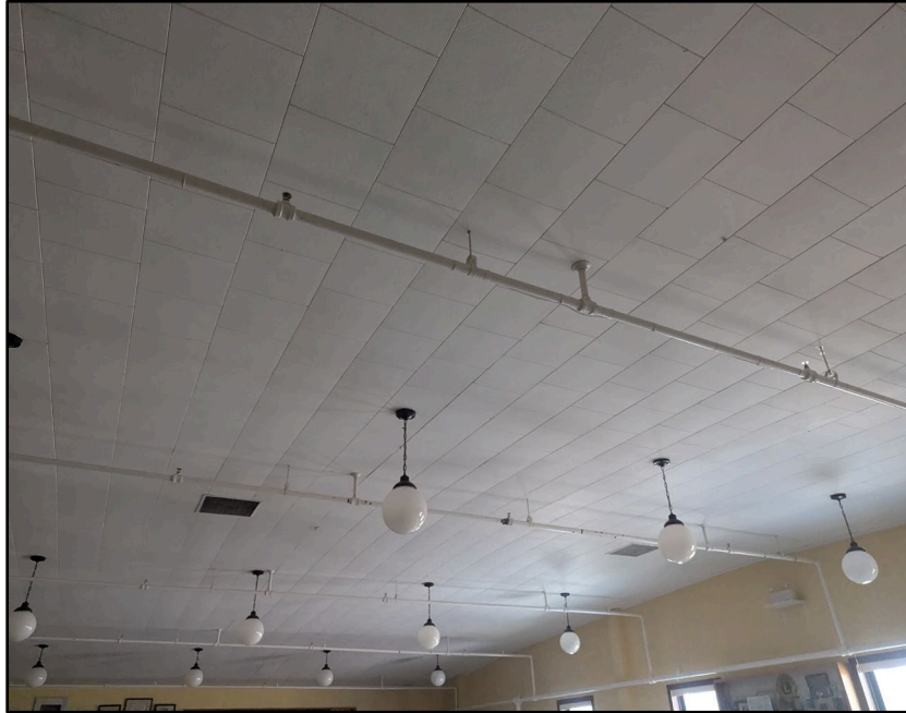
Photo 28: Tube Radiant Heater
