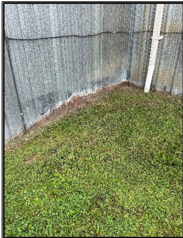
Photo 4: Exterior cladding with visible rusting.
